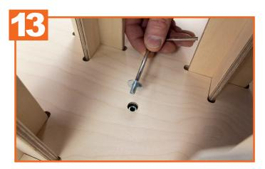
Apply thread locker again and connect screw G (with washer) to the thread.
