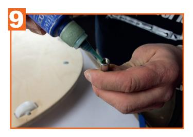
Put thread locker into the thread
